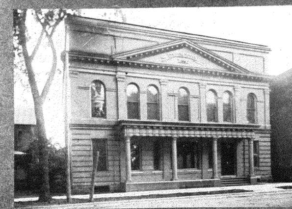
ST. MICHAEL HOSPITAL, WATER WORKS PLANT, MASONIC TEMPLE, STEVENS POINT, WIS.
